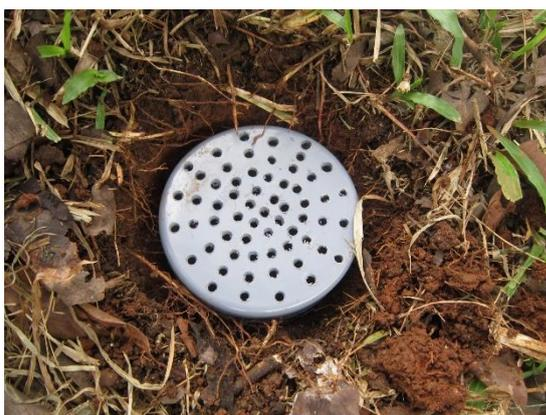
Gambar 7. Hasil lubang resapan biopori
