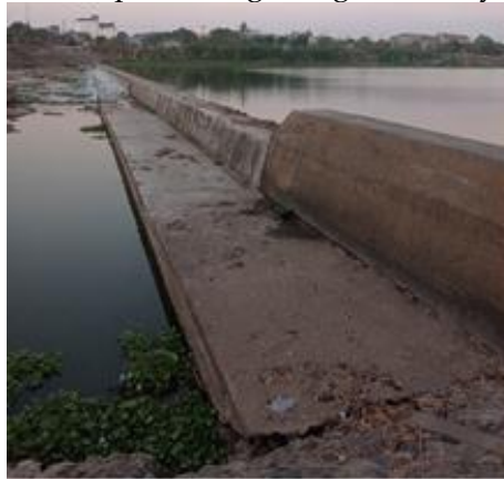
Gambar. Model bangunan groundsill
